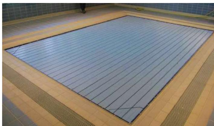
*Automatic movable floor is used to adjust the level of water to each activity the swimming pool may offer.*
